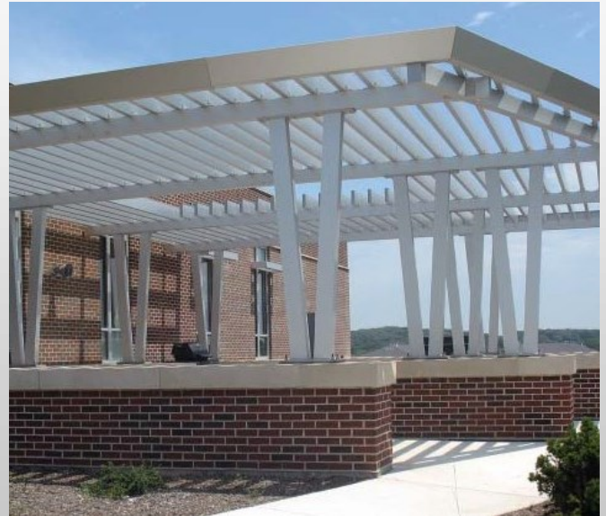
The custom sun control offers protection from the sun for resident firefighters and the public in this outdoor gathering.
